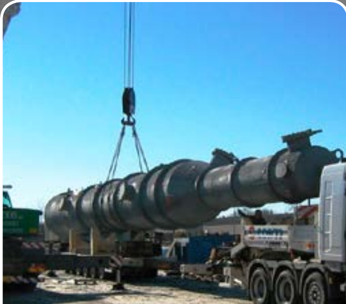
Client/User: ENI SPA / SANNAZZARO DE BURGONDI - ITALY Size/Weight/Design Pressure: ID. 2200/1300 x TL.@TL. 23220 / 31200 Kg / 4,2 Bar.g Material: ASTM A516 GR.60
