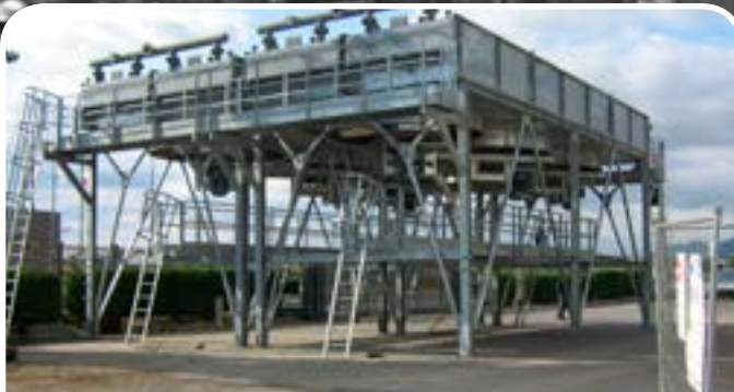
Client/User: FRIGOTECNICA / OVED ZAR - ENI TUNISIA BV API661 Type/Plot Plan/Weight/Design Pressure: PLUG / 10800x12500 / 55000 Kg / 30 Bar.g Tube Type/Material: EMBEDDED Fin Tubes / ASTM A334 Gr.6
